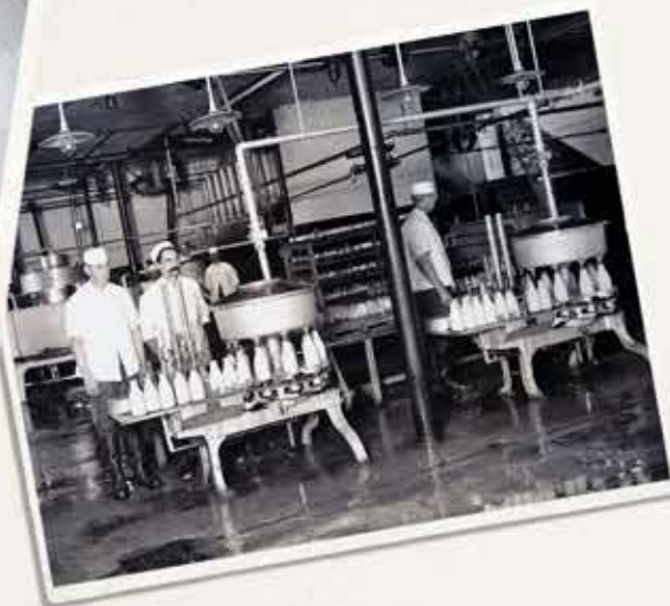
Bowman Dairy Production Facility
