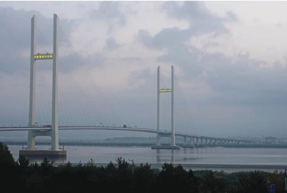
The China-North Korea Yalu River Bridge is seen from Dandong, China, at the border between the two countries.
