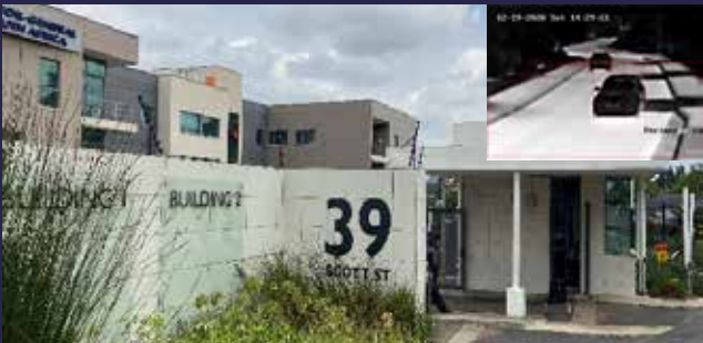
Office Building Entrance
