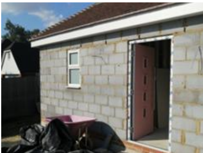
Rubie's wet room under construction
