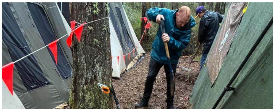
Digging a drain in the rain
