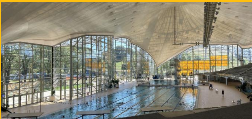
Munich Olympic pool
